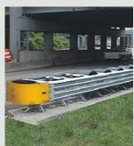
The QuadGuard Elite System, besides being self-restoring after most design impacts, is designed to withstand multiple impacts without the need to replace the HDPE cylinders. After each impact, maintenance crews should measure the shorter diameter of the last cylinder (closest to the backup). When this diameter is reduced from its original 815 mm (32") to 660 mm (26") or less, all of the HDPE cylinders will need to be replaced
