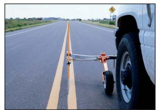
Using the Video Guidance System accessory while restriping a straight stretch, the operator watches the video screen and lines up the indicator along the line to an infinite distance, eliminating the need for frequent corrections.
