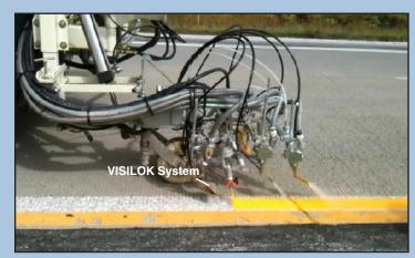
The VISILOK System is an easy modification by spraying VISILOK into the paint stream.
